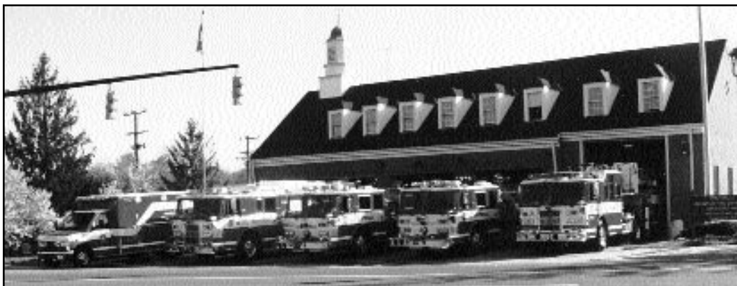
The firehouse today is no longer capable of accommodating the community's short and long term needs for quality fire, rescue and emergency medical services
